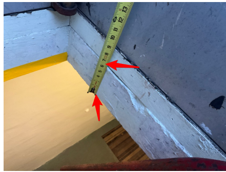
Concrete roof deck
