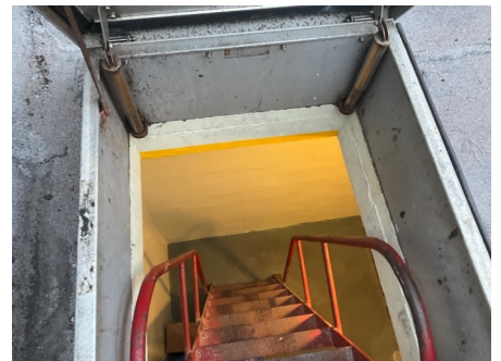
Concrete roof deck
