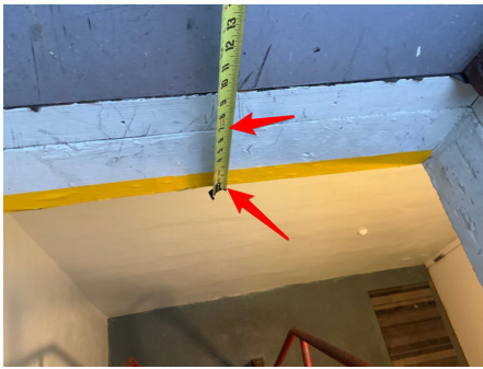
Concrete roof deck
