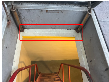
Concrete roof deck
